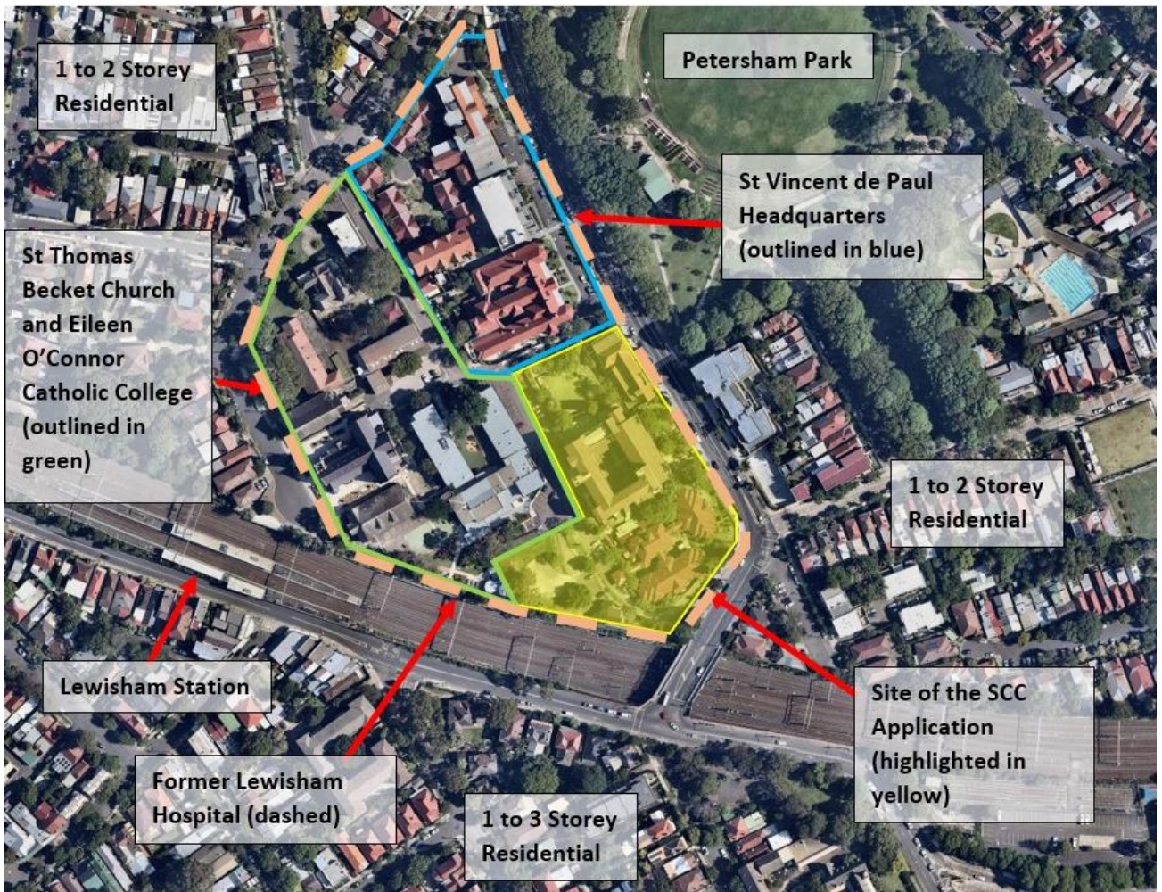
Figure 2 – Aerial photo of the surrounding area (Source: Nearmaps)
